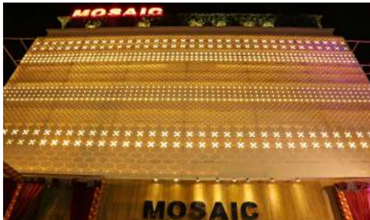
Mosaic Banquet Hall in New Delhi wears a stylish and durable façade made from DuPont™ Corian®, incorporating an effective lighting design; Corian Fabrication & Photo courtesy: Oystra Concepts Pvt. Ltd.
